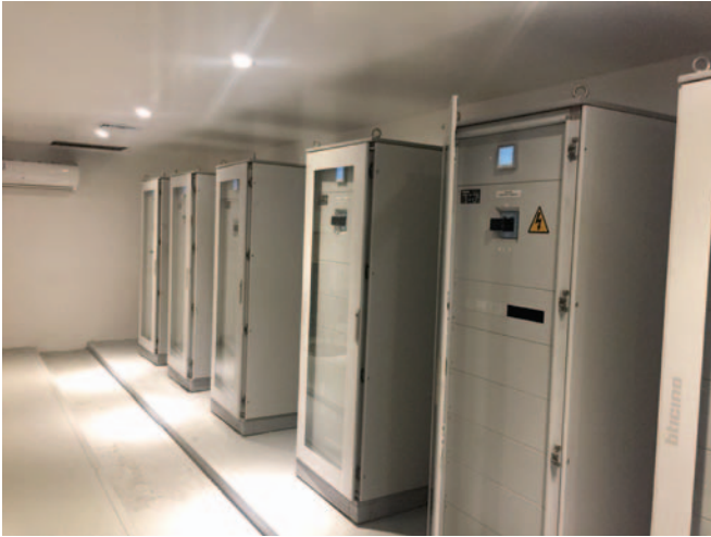
Medium voltage (13.8 kV) to low voltage transformer vault.
